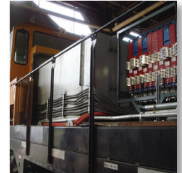
Installation on locomotive
