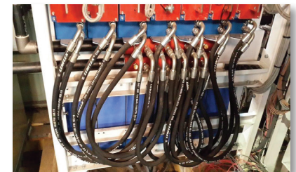
Modules are liquid-cooled using cooling hoses and manifolds.
